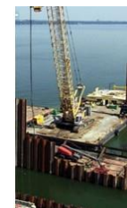
Figure 2. Project Execution in Randle Reef, Hamilton Harbour (Lake Ontario)
